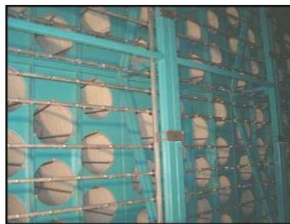
Nozzle Array Erection with Piping Interconnection at Ferrera Erboگونه
