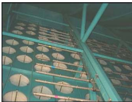
Nozzle Array Erection with Piping Interconnection at Ferrera Erboگونه
