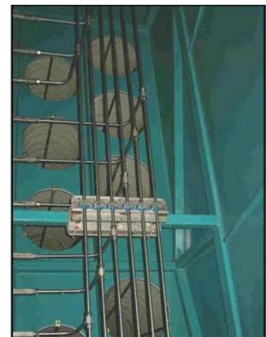
Nozzle Array Erection with Piping Interconnection at Ferrera Erboگونه
